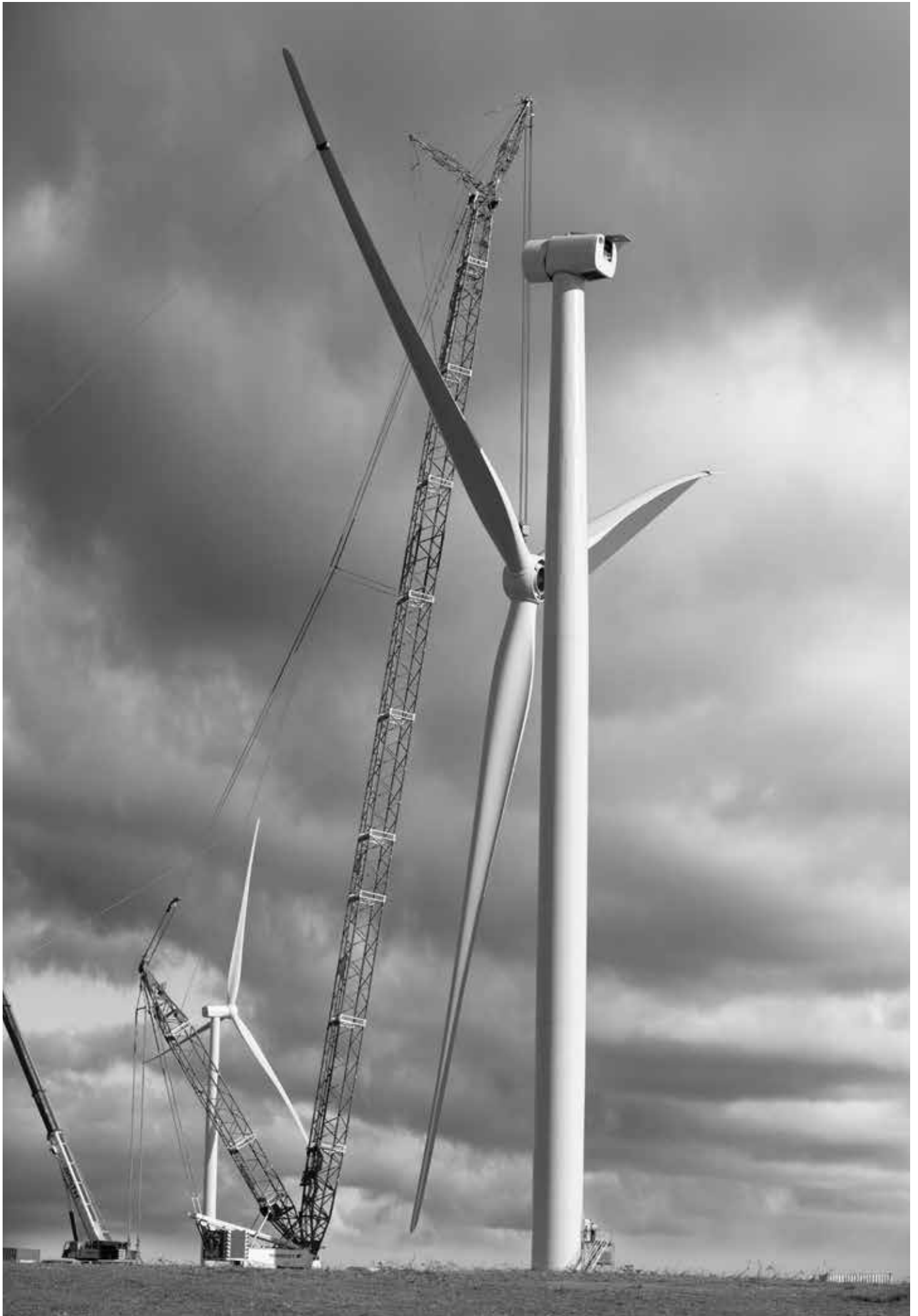
Erecting one of Waipipi Wind Farm's 31 turbines 7 kilometres southeast of Patea. The blade tip reaches 160 metres from the ground
