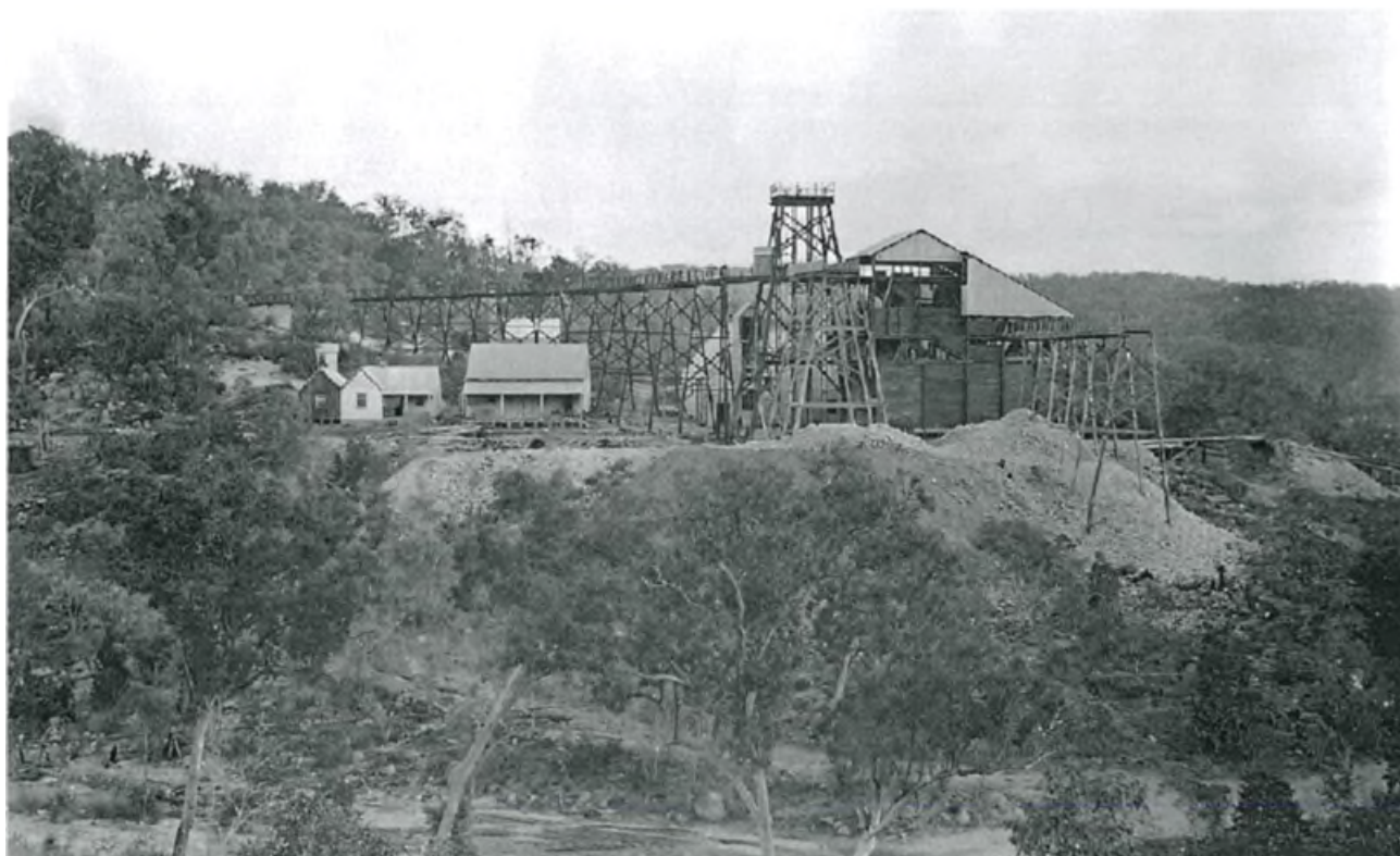
Figure 6 - King Conrad Shaft, Historic Photograph
