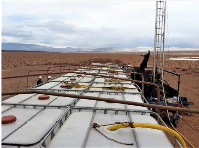
Pumping Brines - Kachi
