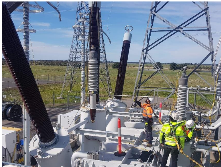
Wind farm near Hamilton, Victoria - 132KV bushing replacement on 500kV/132KV transformer being undertaken by STE Solutions
