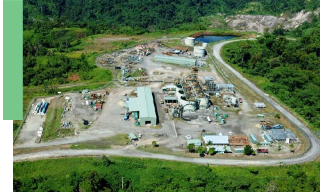
GOLD RIDGE GOLD PLANT ON GUADALCANAL
