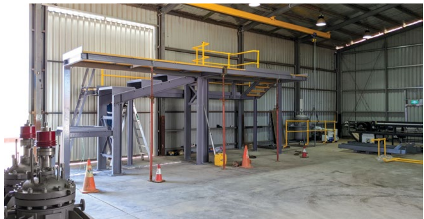
Figure 1 – Pilot Plant Progress Update – Steelworks being installed
