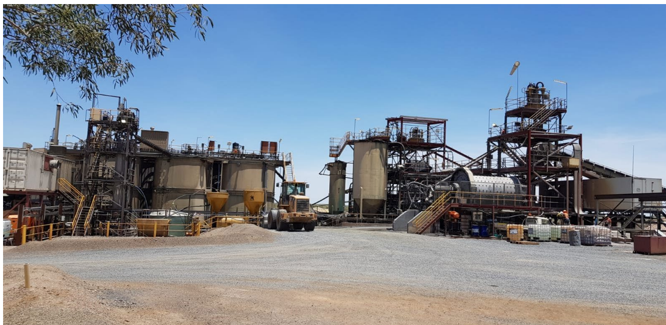
Figure 1 - Lorena Gold Mine CIL Processing Plant starting Processing Agate Creek Ore
