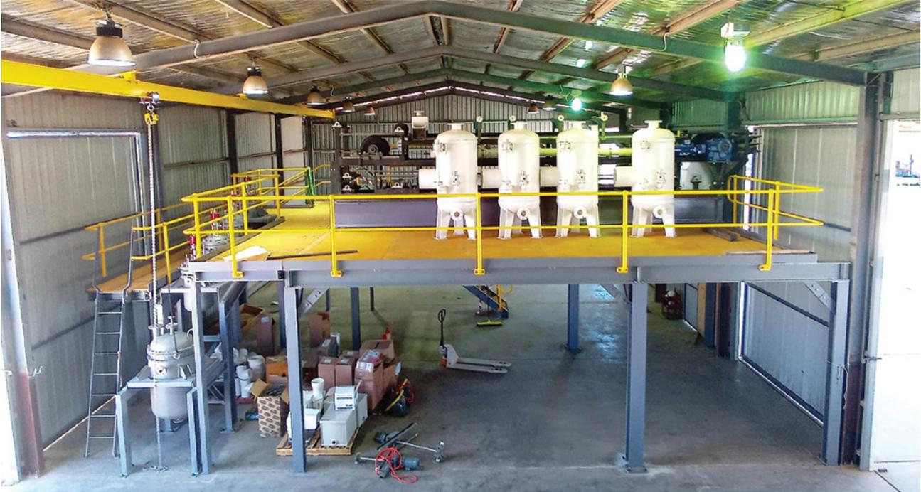
Figure 2 – Pilot Plant – installed autoclave reactors in foreground
