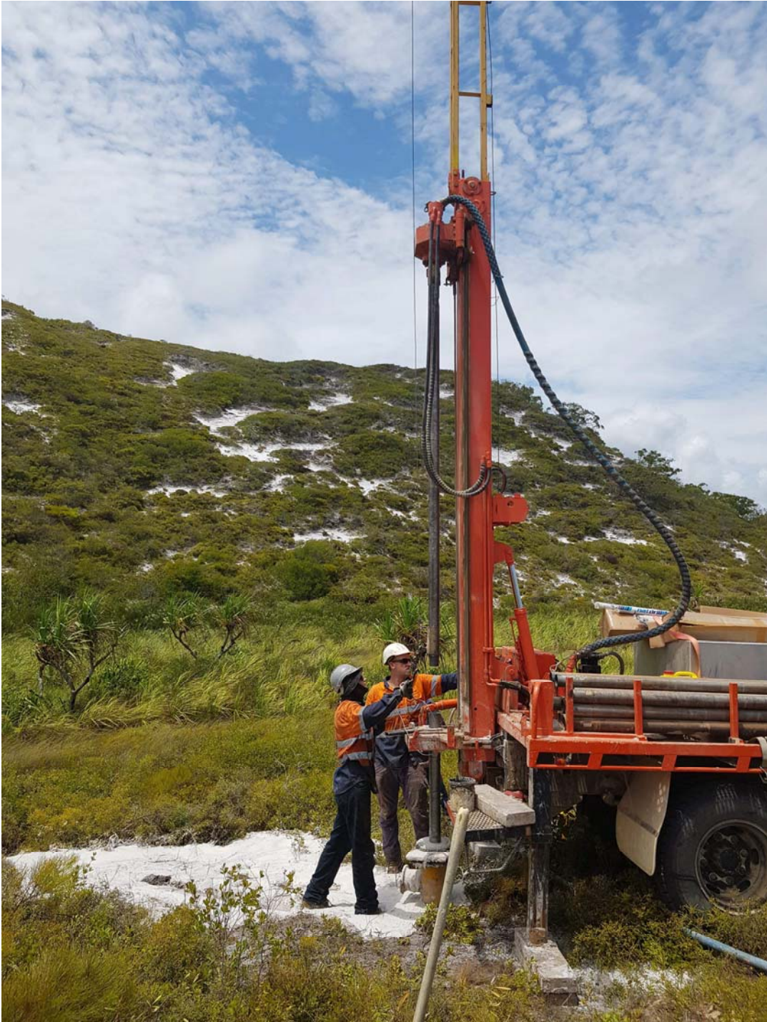
Figure 2: Groundwater bore drilling on site
