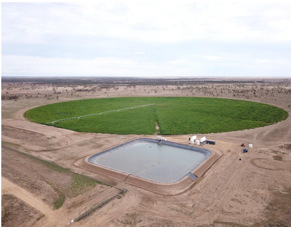
Figure 4 – Aerial view of Glenaras Water Management Project.
