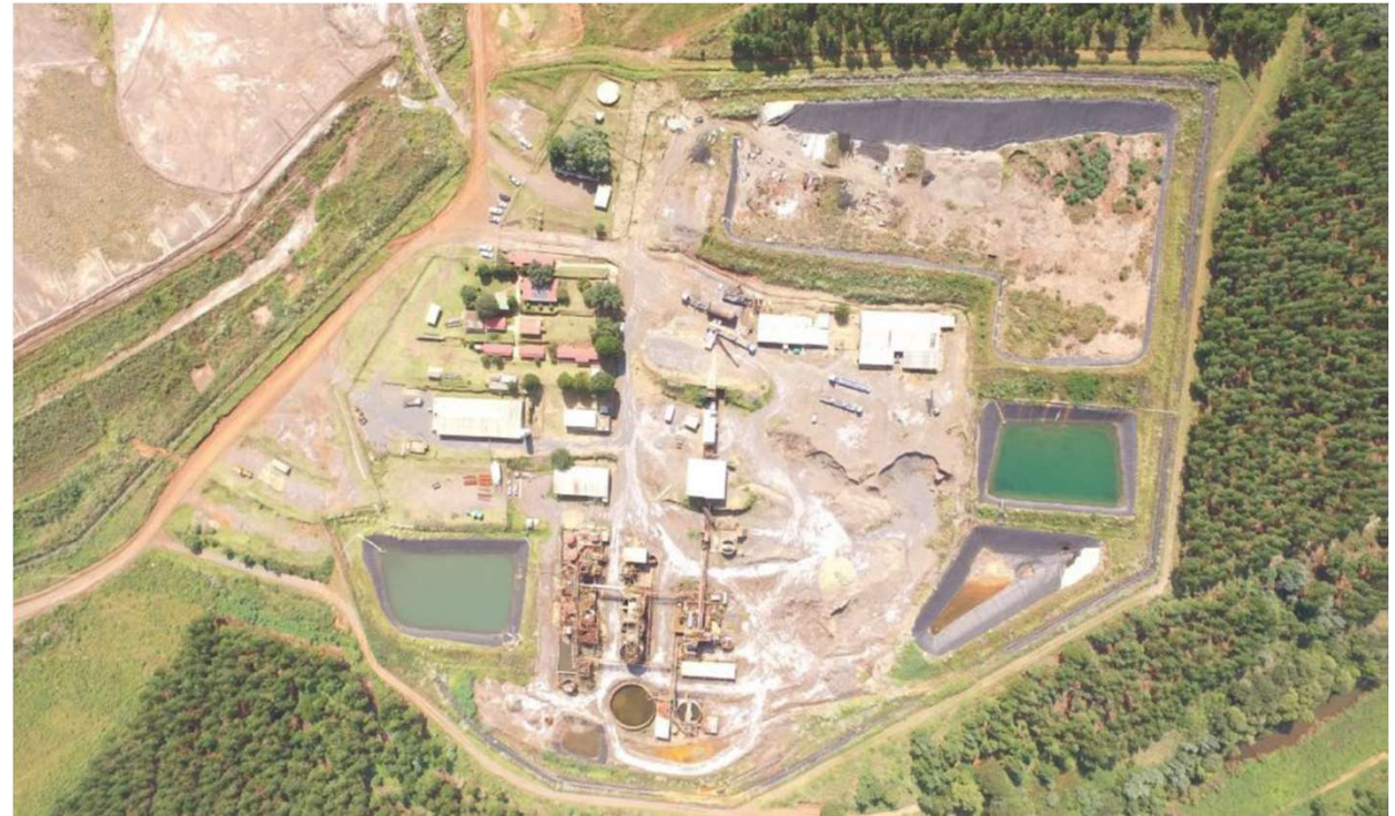
TGME GOLD PLANT FOOTPRINT- Tailing Storage Facility (TSF), admin building, machinery shed, water, and Power onsite
