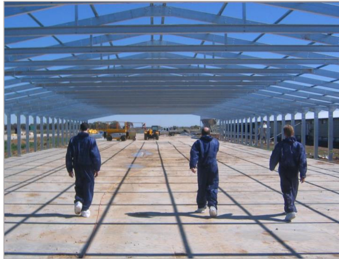
Poultry shed construction, Griffith - New South Wales, August 2006.
