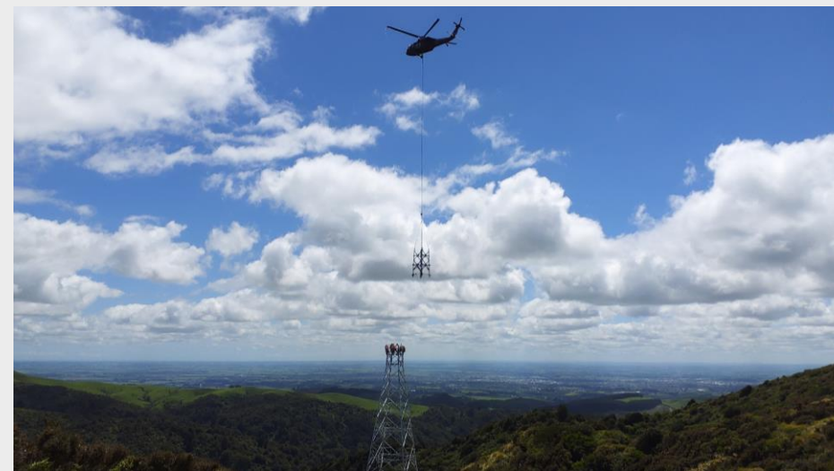
Transmission tower construction
