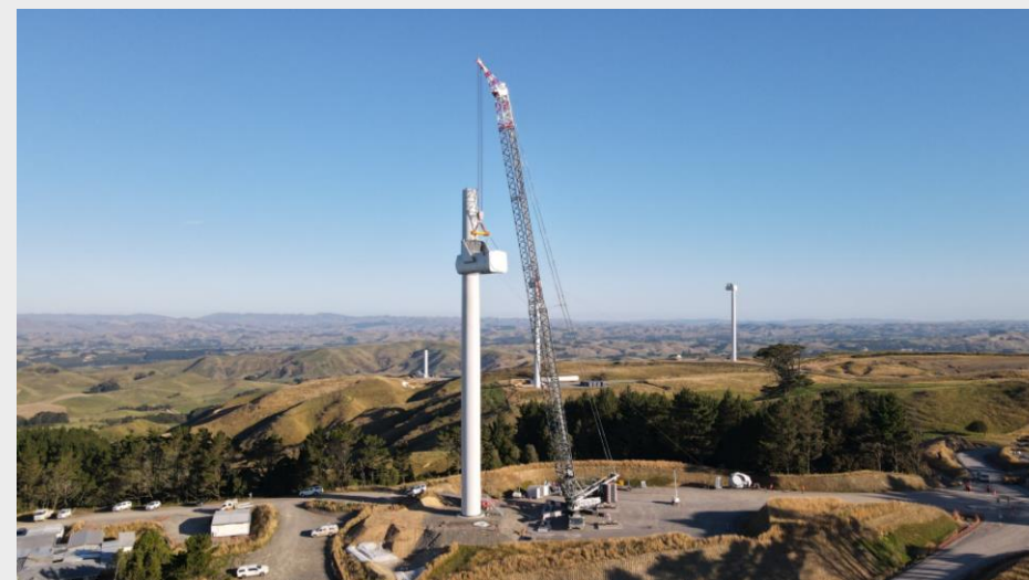
Nacelle installation
