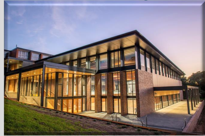
San Clemente High School, Mayfield NSW Won the Master Builders Association Newcastle Excellence in Building Award
