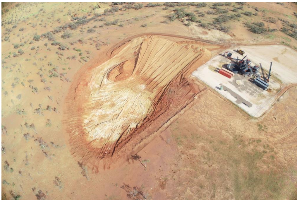
Pit excavation adjacent to process plant
