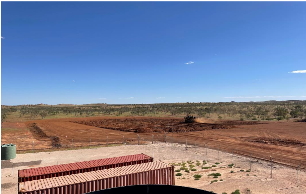
Initial pit area overburden removal
