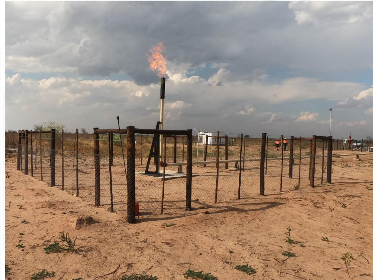
Gas Production well in the Lesedi project area
