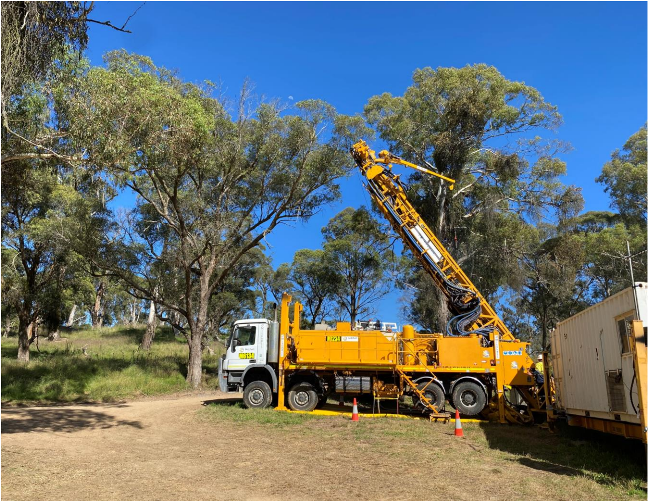
Figure 3. One of the two surface diamond drill rigs recently mobilised to the Dargues site to target down dip and strike extensions to the MRE.
