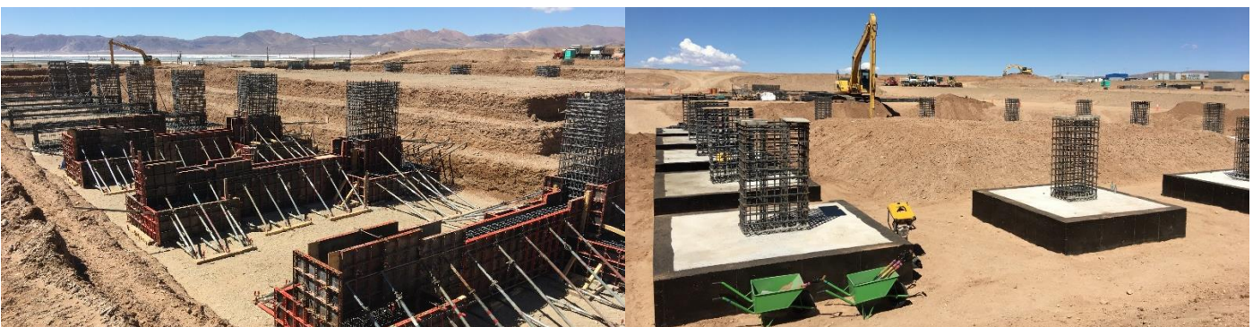
Note: new carbonation plant and soda ash facility footings
