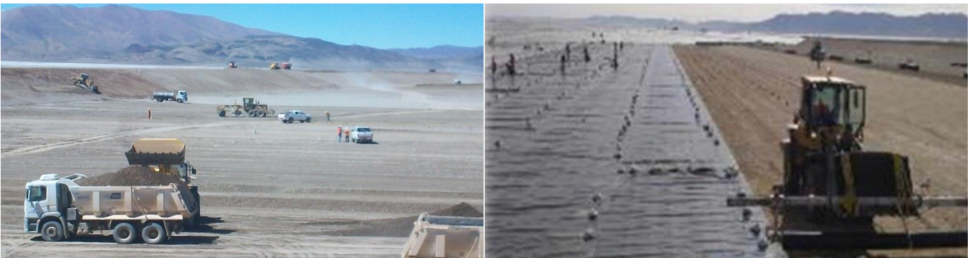
Note: additional ponds under construction
