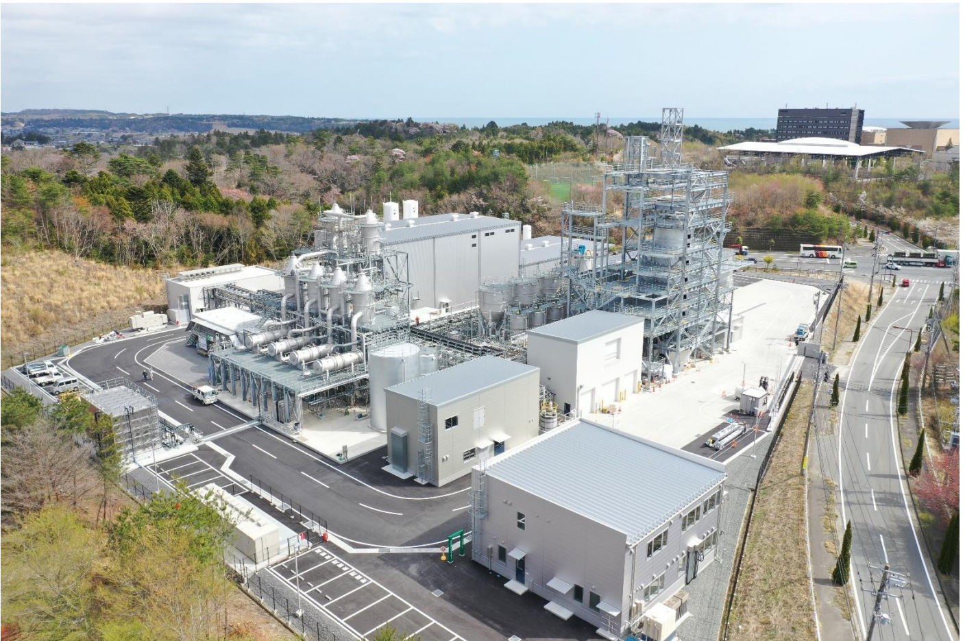
Aerial view of the Naraha Lithium Hydroxide Plant construction site
