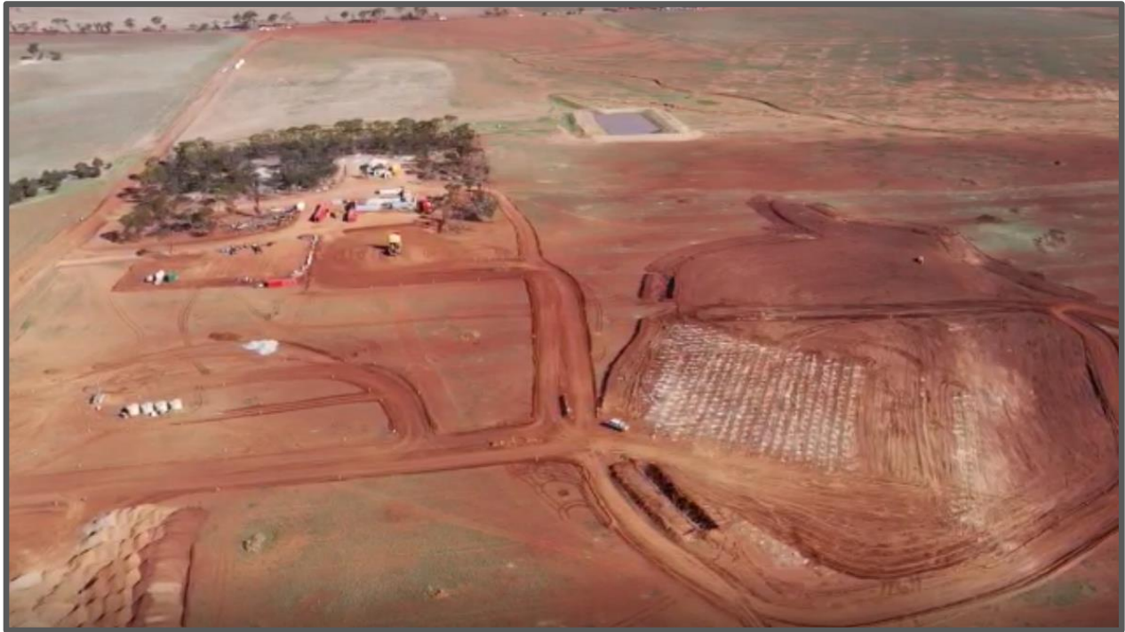
Figure 7: Tampia open pit commencement looking south
