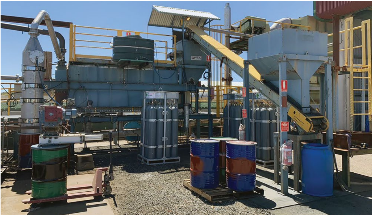
Figure 4 – Calcine circuit operations (ANERGY Bunbury)
