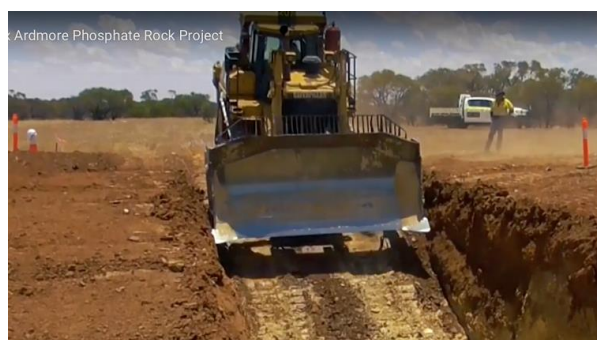
Dozer operation at Ardmore
