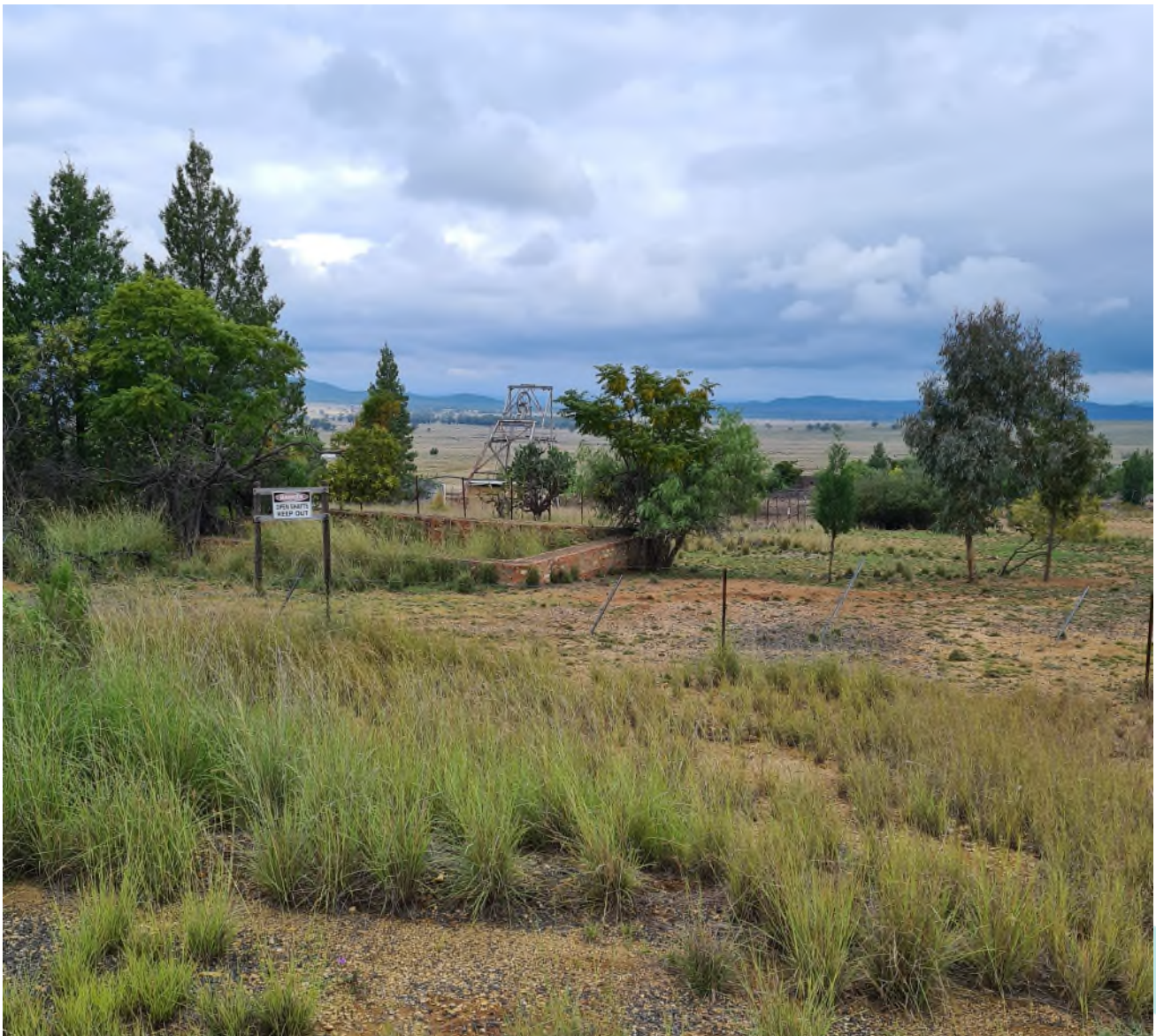
Figure 1 – Image from recent Silver Spur site visit
