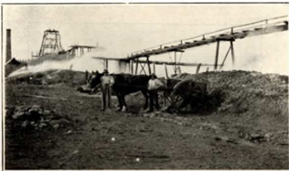
Open-air roasting in kilns, Silver Spur Mine (above), General view of township and surrounding districts, Silver Spur (right). GSQ Publication 243, 1913. Geology and Mineral Resources of The Stanthorpe, Ballandean And Wallangarra Districts (with Notes On The Silver Spur Mine, Texas). Report CR055399. From GSQ Open Data Portal https://geoscience.data.qld.gov.au/
