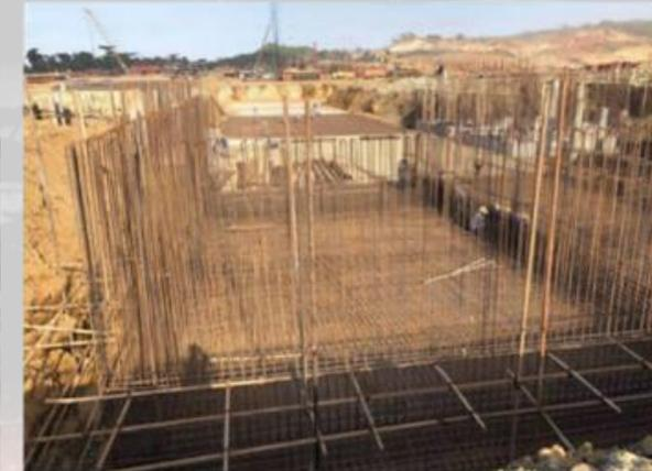
Area for electrostatic precipitator
