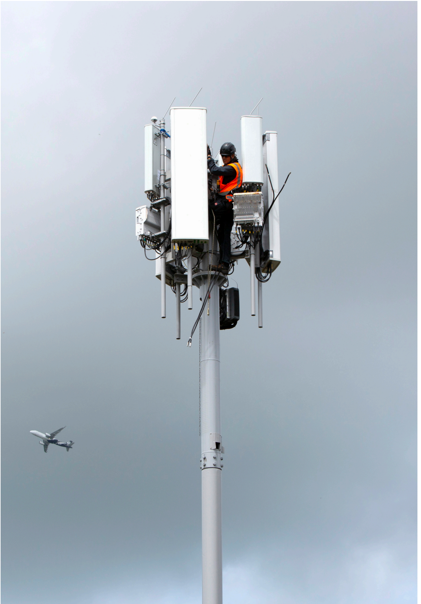
Vodafone 5G tower installation, Māngere, Auckland
