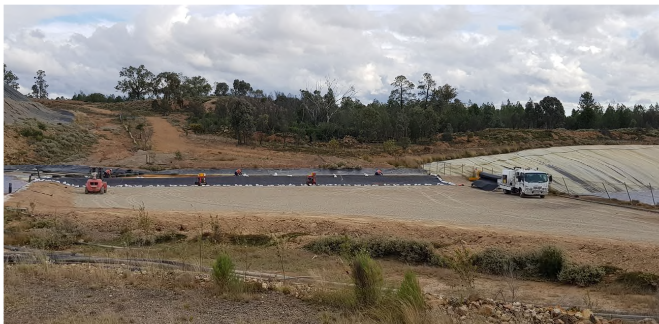
Figure 11 – Installation of heavy duty plastic protective sheeting being undertaken at Texas Silver Project in preparation for installation of Thomson provided evaporators near Terminal Dam
