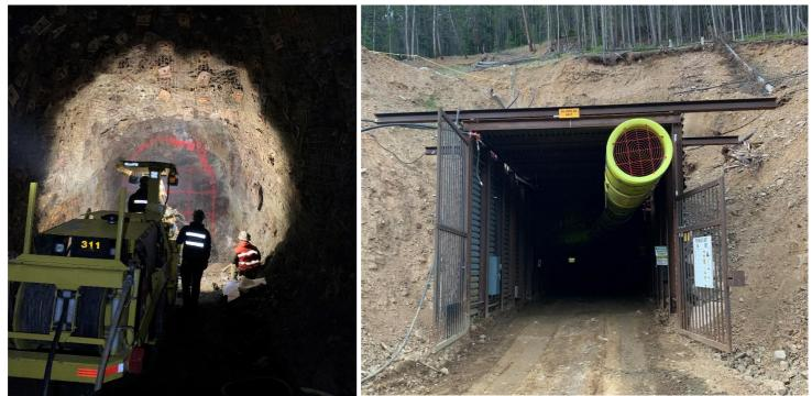
Figures 2 and 3: Jumbo drill rig at development face and newly upgraded ventilation at portal
