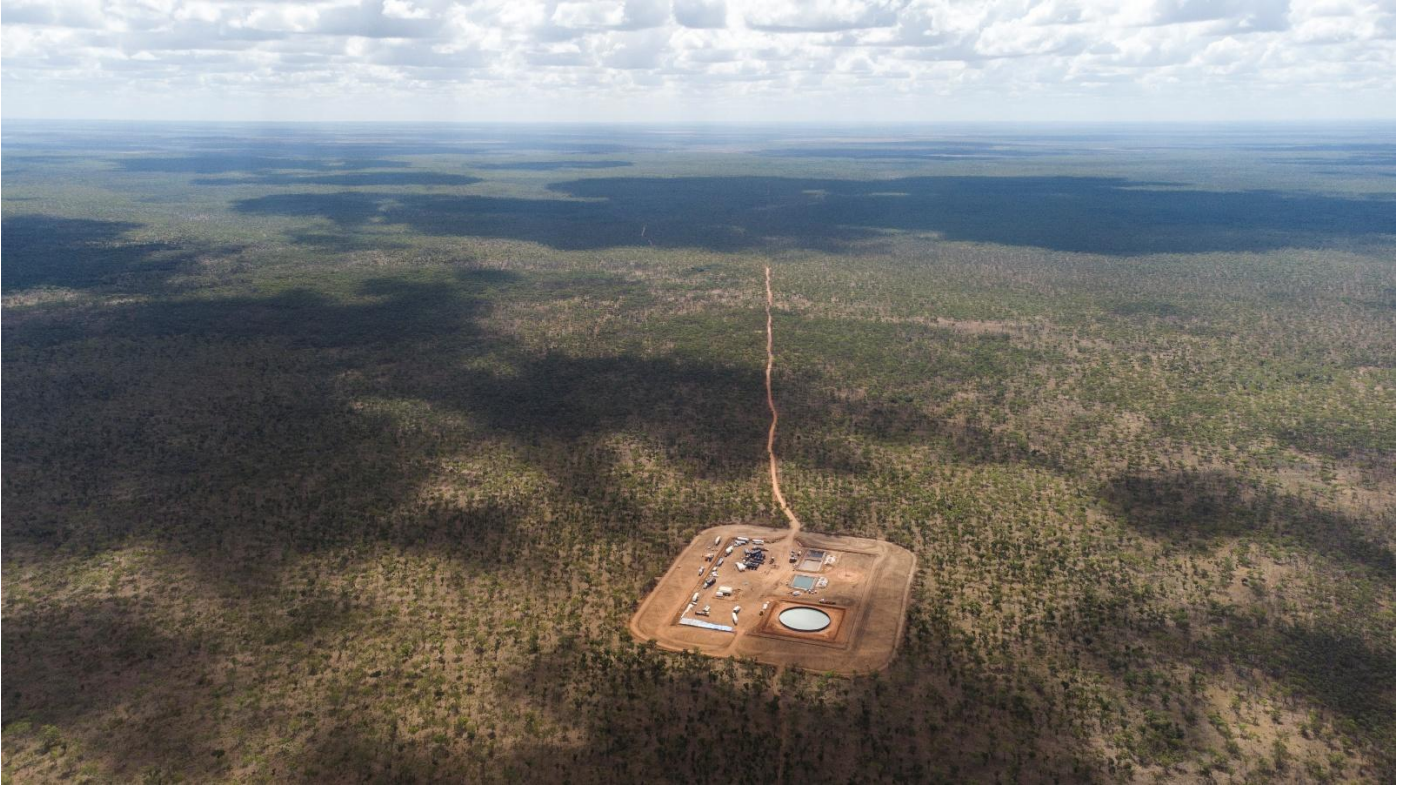
Carpentaria-1 located in EP187 during vertical fracture stimulation operations
