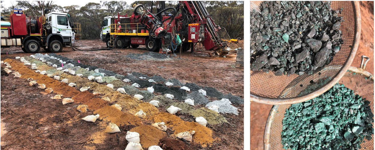
Figure 3 – Drill rig at HWRC003 (left) with sieved chips showing contrast between mineralised structure and fuchsite halo (right)
