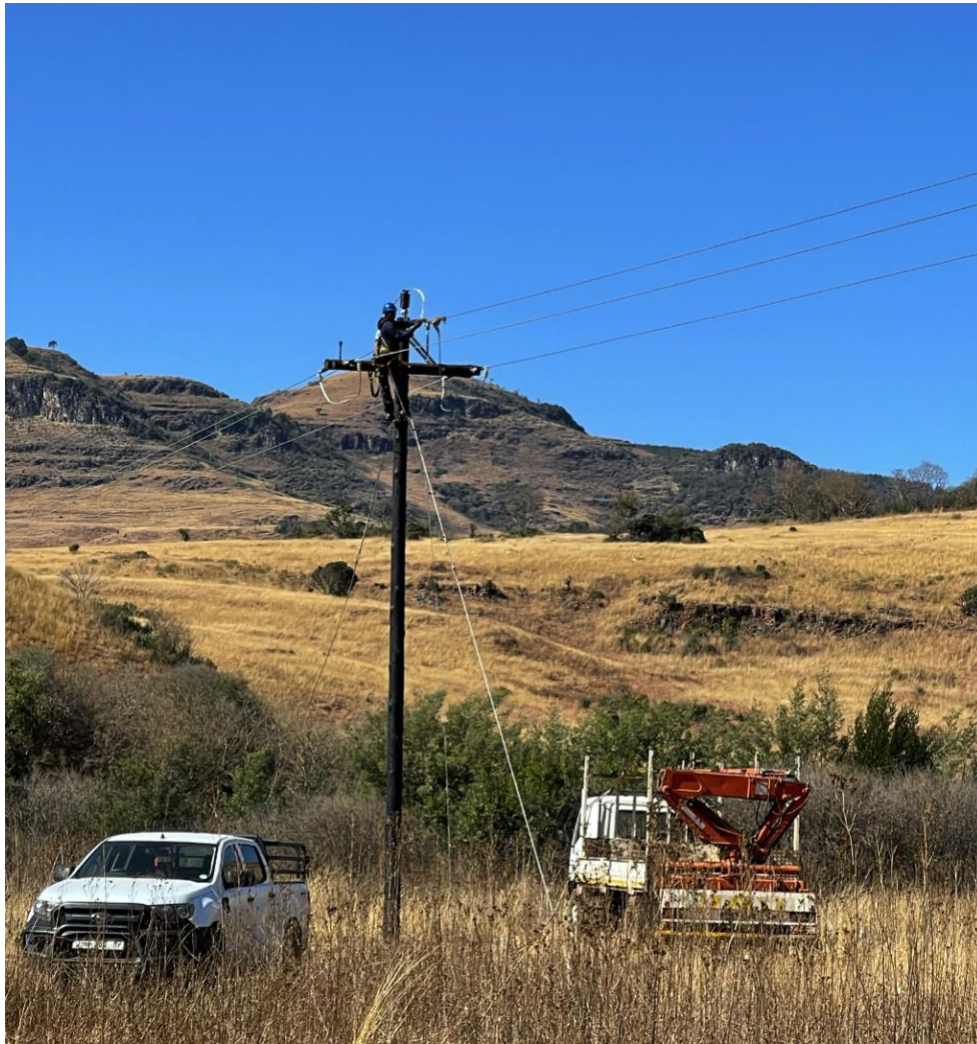
Figure 2 – Government funded new power line installation across the Northern section of our Mining Rights (close to Vaalhoek and Frankfort mines). The powerline will add to the required capacity for the new gold plant and extends from north to south over 20 km within the current Mining Rights area.
