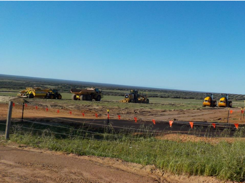
Waitsia Stage 2 Clearing, Western Australia
