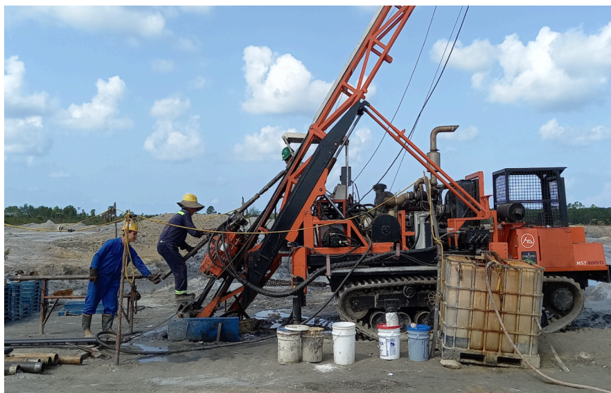
Drilling at La Demajagua
