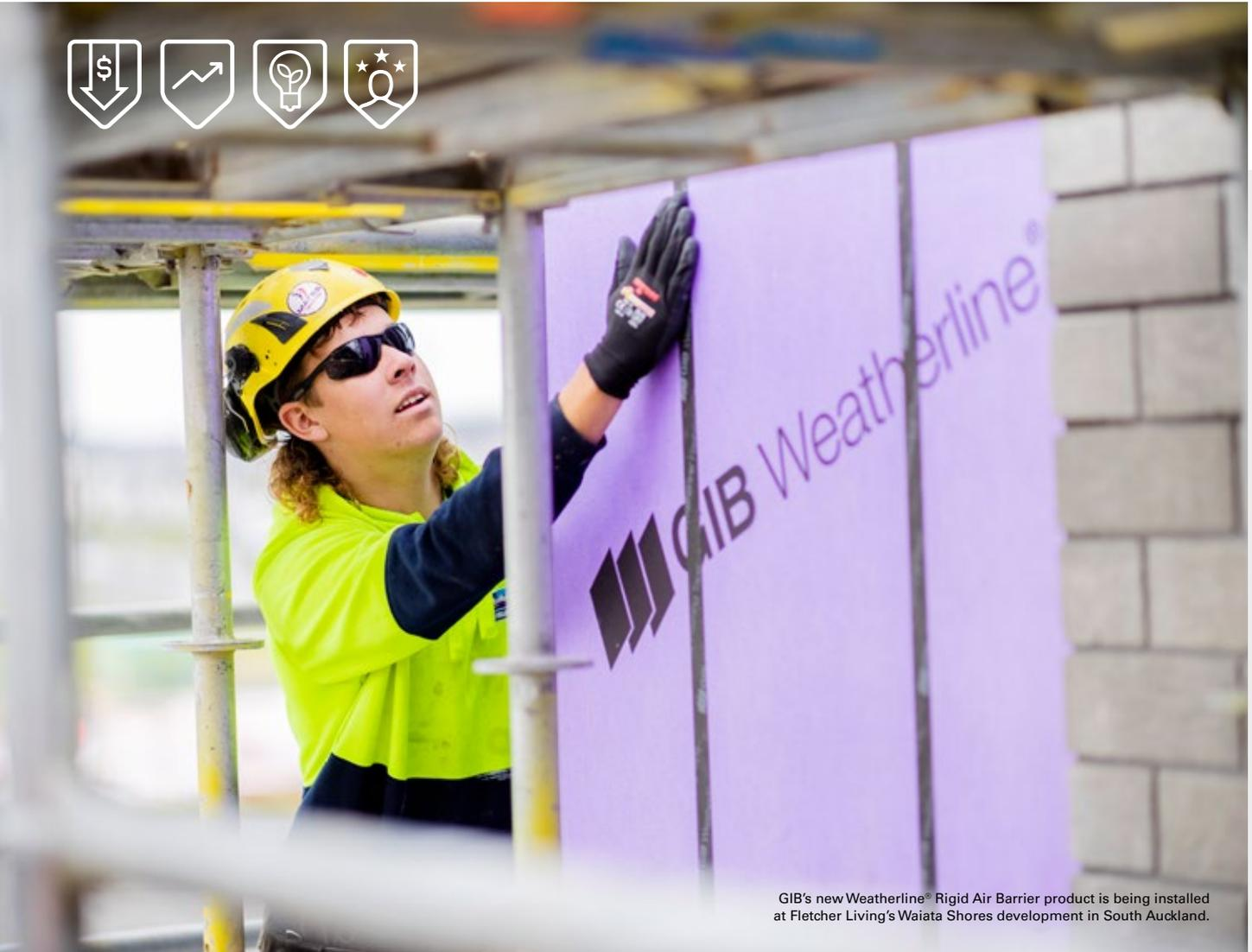
GIB's new Weatherline® Rigid Air Barrier product is being installed at Fletcher Living's Waiaata Shores development in South Auckland.
