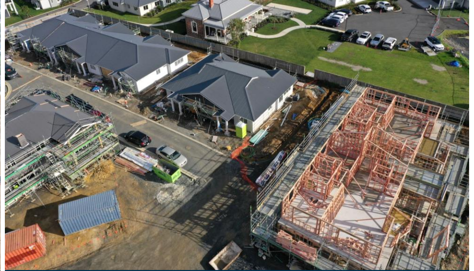
Summerset at Monterey Park (Hobsonville, Auckland)
