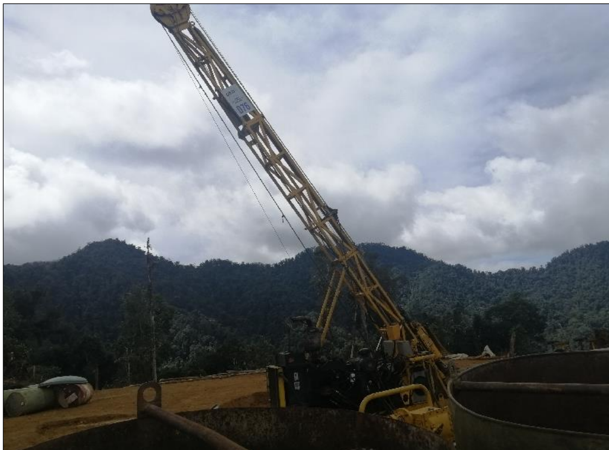
Figure 2. Diamond drill rig set up on MW001 (Mt Wipi)
