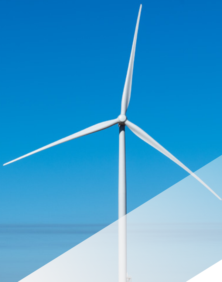
Badgingarra Wind Farm, Western Australia
