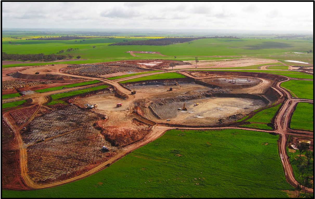
Figure 7: Tampia Open Pit commencement, looking North, July 2021
