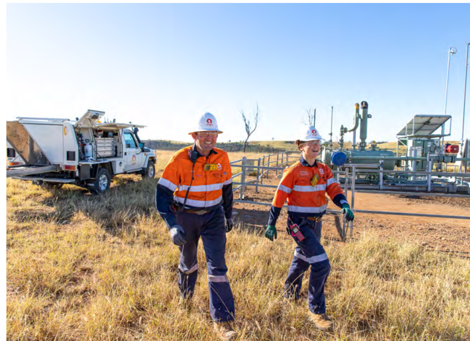
Origin employees undertaking well maintenance in Spring Gully.
