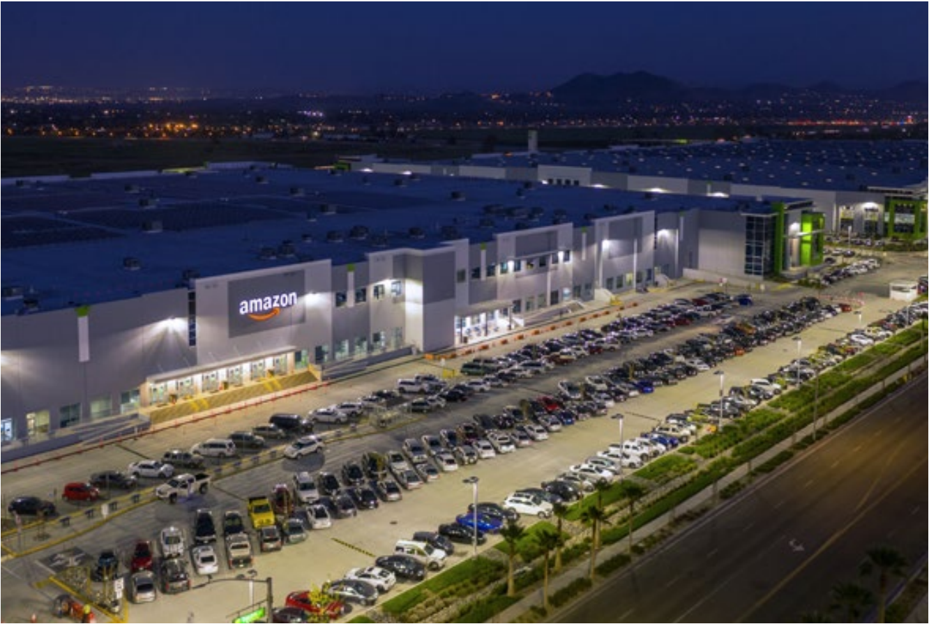
Goodman Commerce Center Eastvale, Los Angeles, USA.
