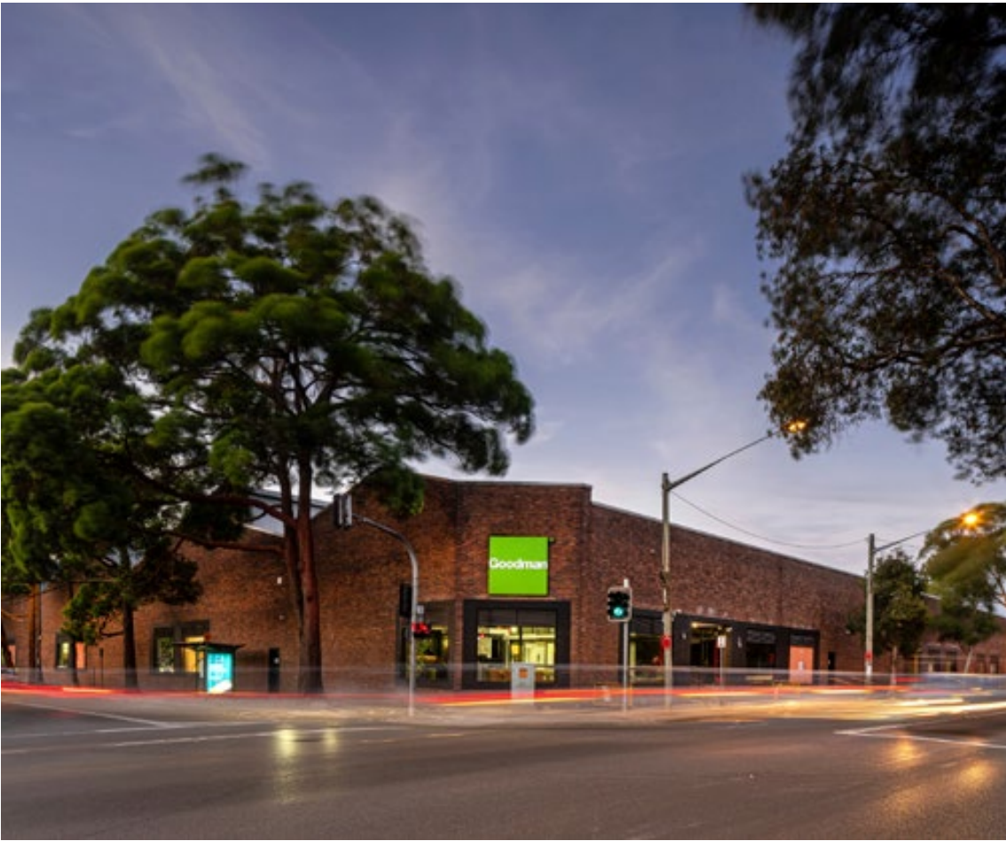
Alexandria Industrial Estate, Sydney, Australia
