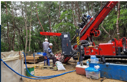
Drilling at Nettle, Deokon Project.
