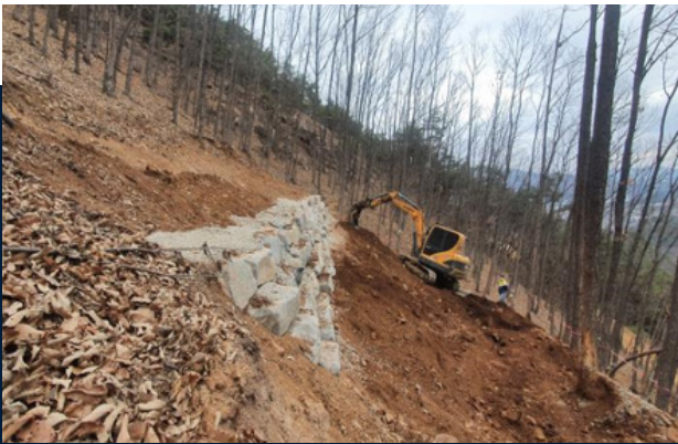
Weolyu track rehabilitation on government forest land.
