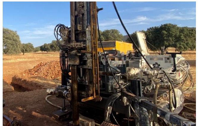
Figure 2. Geotechnical drilling was 50% complete at the end of the quarter
