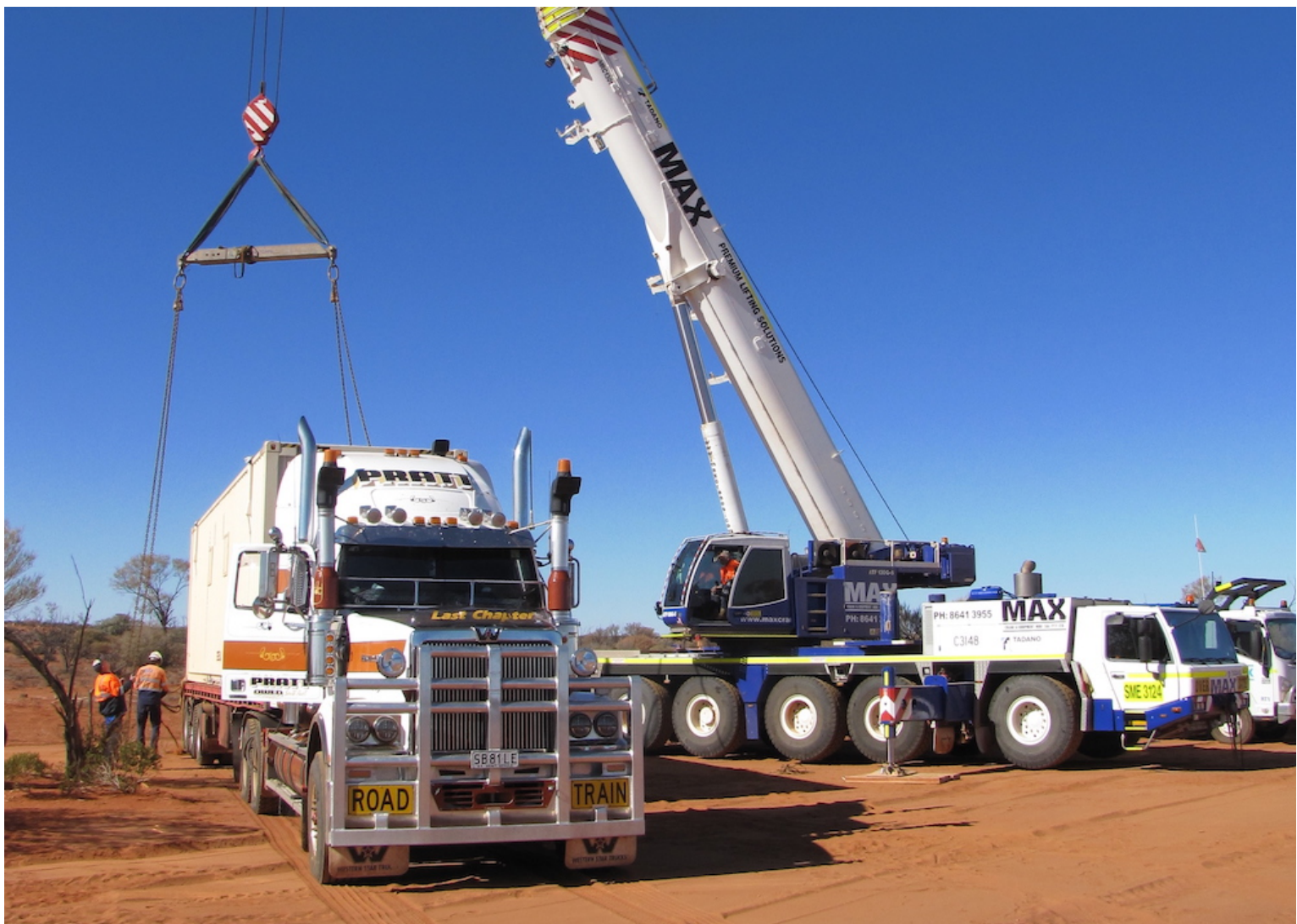
Figure 7: Components of camp being unloaded at Aurora Tank from road train during FY21
