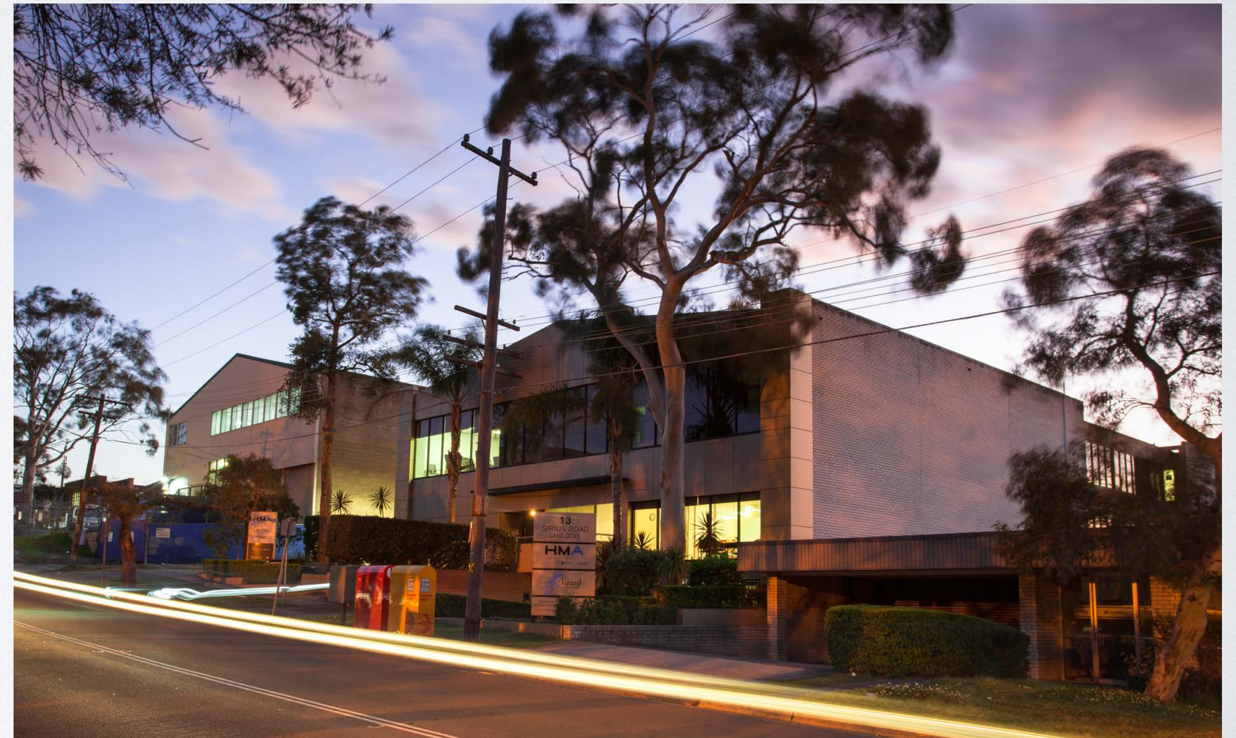
13 Sirius Road, LANE COVE NSW
