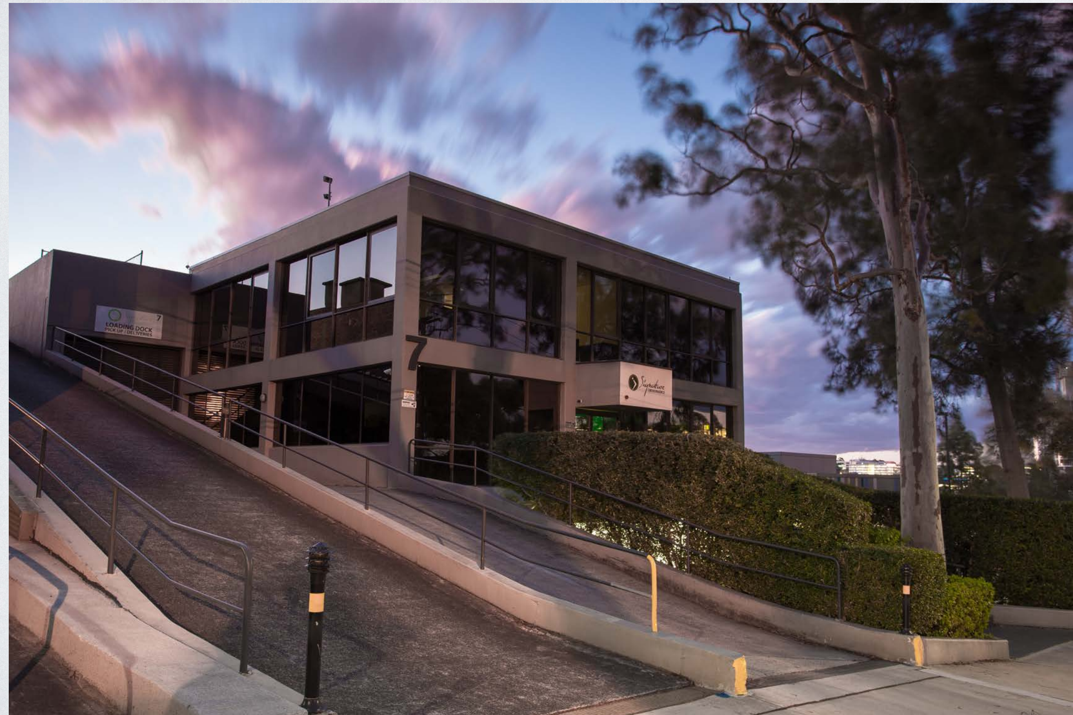
7 Sirius Road, LANE COVE NSW
