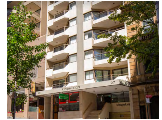
Metro Apartments on King 27-29 King Street Darling Harbour, Sydney NSW 2000 T: 61 2 9290 9200
