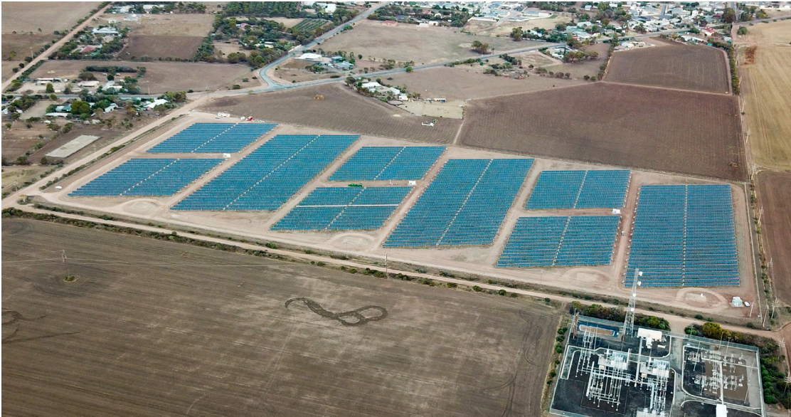
Image: Kadina Solar Farm designed and constructed by MPower. MPower has received the final milestone payment for the project.
