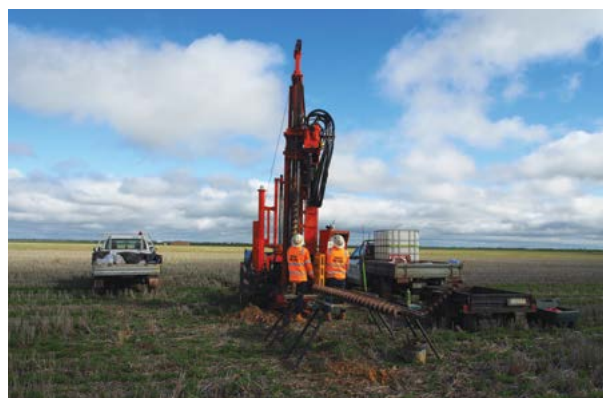
Astron Donald Project site geotechnical drilling (2021)
