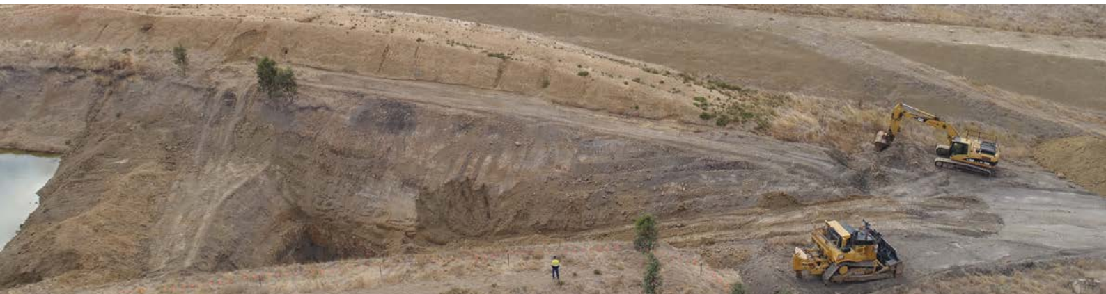
Donald Mineral Sands' Project excavation test pit.
