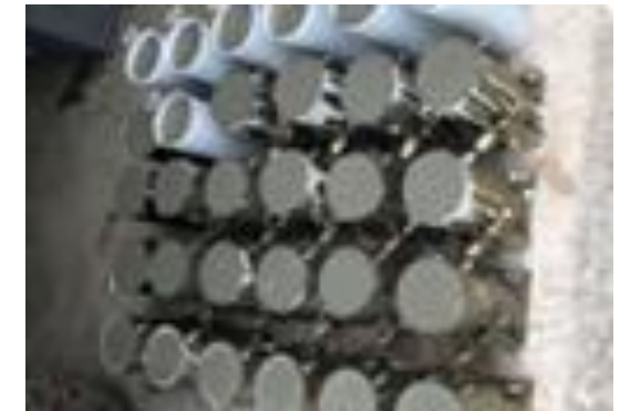
Only 1kg in 3 tonnes of concrete required
