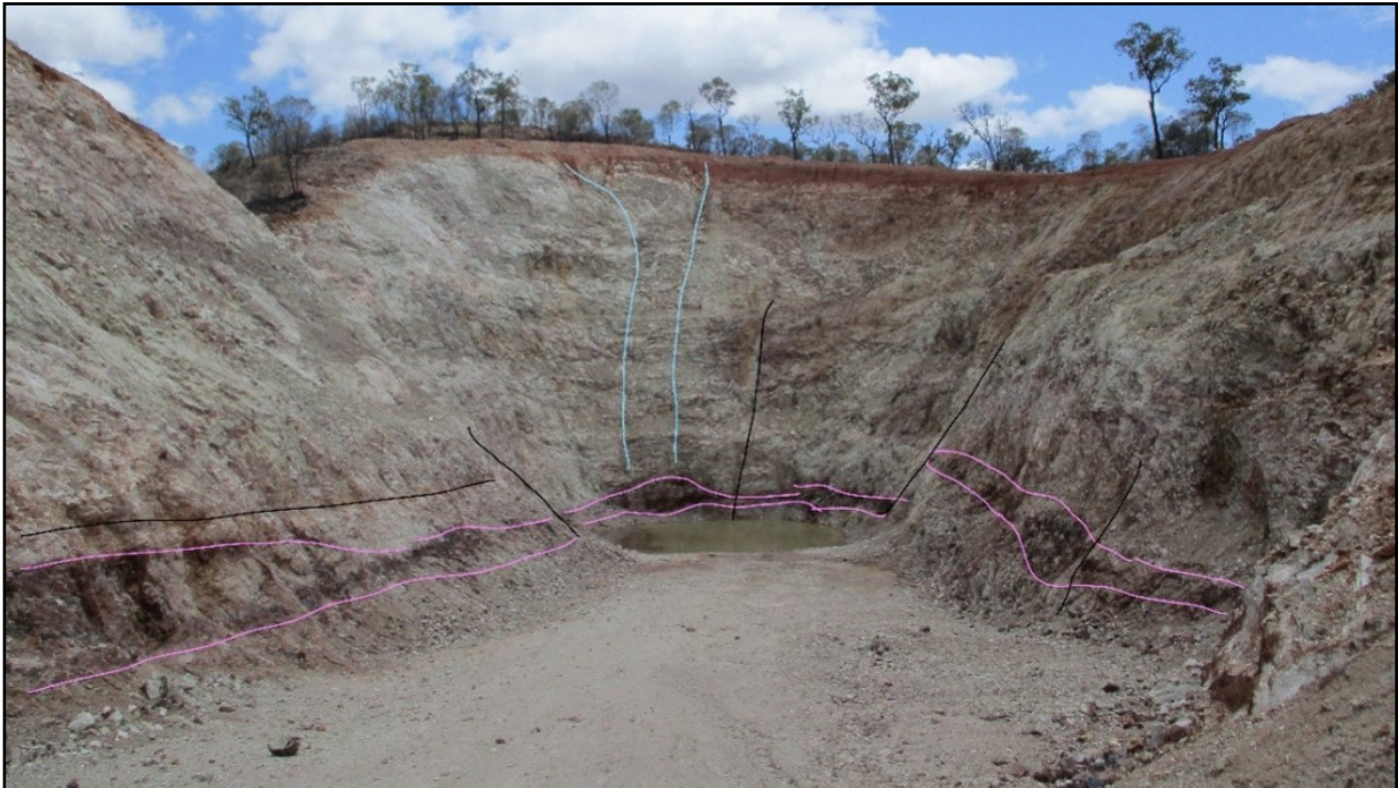
Figure 5: Sherwood Open Pit, looking NE, showing shallow dipping rhyolites comprising breccias (pink outline) along a hanging-wall thrust contact (black line).
