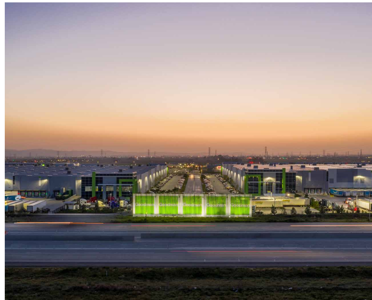
Goodman Commerce Center Eastvale, Los Angeles, USA
