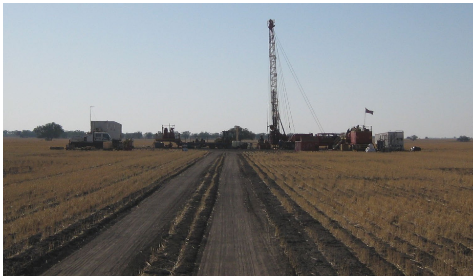
Myall Creek #04 Workover – Dec 2019 (Myall Creek#2 will be similarly set up)
