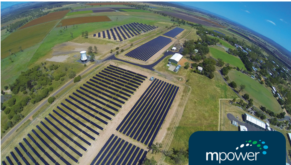
Image: University of Queensland battery storage project designed and constructed by MPower
